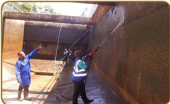
According to Mr Issa Kassim the Production Supervisor at the Plant, apart from removing accumulated sludge and cleaning the walls the process also removes algae that causes foul smell in water.
