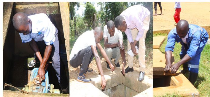
Controls team at work
