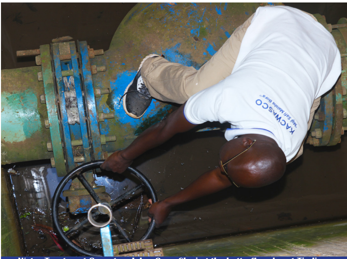
Water Treatment Operator, Jalon Oyoo Closing the butterfly valve at Tindinyo
