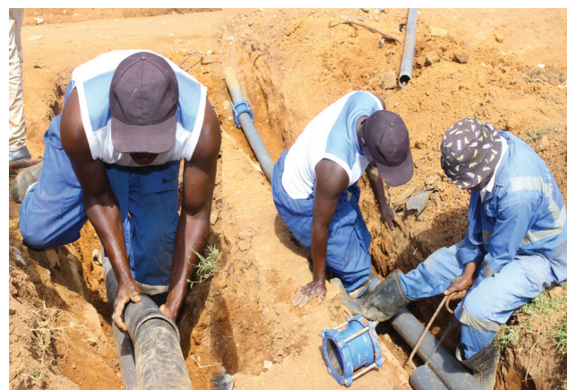
KACWASCO team fixing pipes at Amalemba Estate
