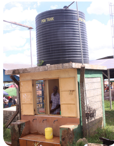
A Water Kiosk at Butere Lower Market
