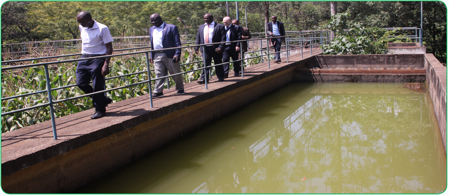
Technical Manager Mr Celcus Shilehwa with a team from MENA water during a field visit at old Kakamega Water Treatment Plant
