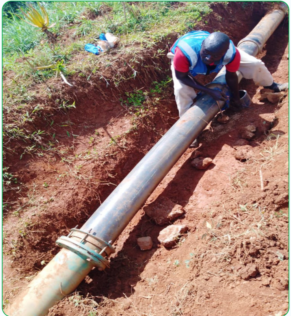
KACWASCO O&M artisan during the pipeline extension exercise
