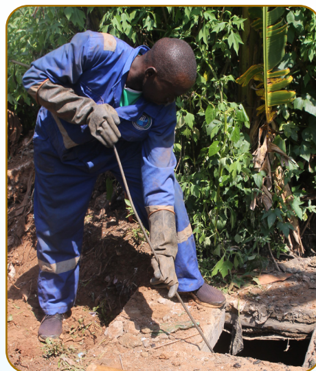
Athanus Masheti Artisan Waste Water unblocking Sewer man hole
